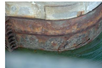
Discontinuity due to fatigue (cyclic loading)
