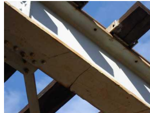
Discontinuity due to fatigue (cyclic loading)
